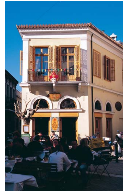
60. Two-storey neoclassical building at Iroon Square (Psyrri).
