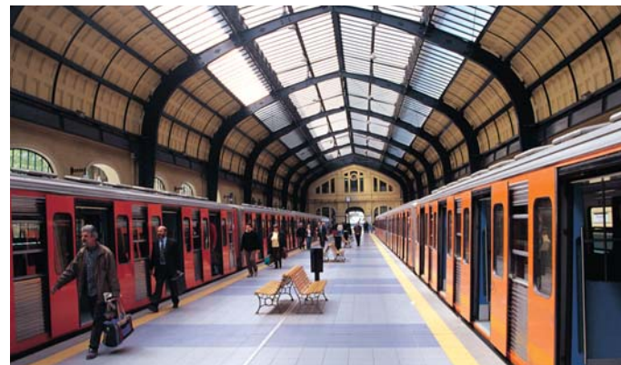
156. The renovated Piraeus metro station.
