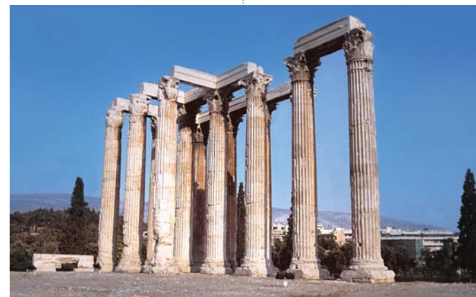
2. Temple of Olympian Zeus: 16 of a total of 104 columns (with a height of 17 metres) have been preserved.
