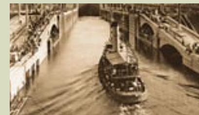
Theodore Roosevelt believed a canal was indispensable to U.S. supremacy at sea, which was secured by the trial lockage in 1913.
